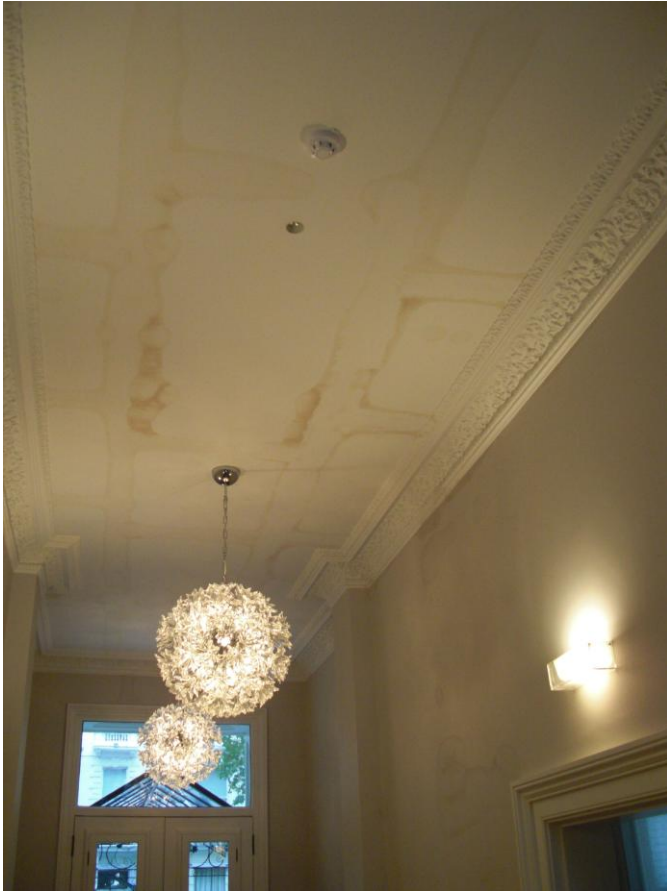
Before: Damp ceiling joists
